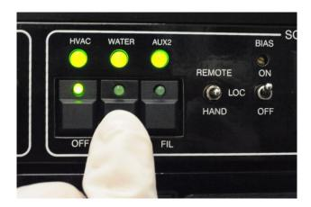
Step 9: Move the Remote/Loc/Hand toggle to Remote.
